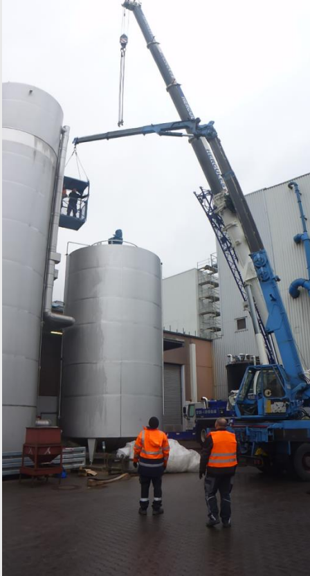
Construction of the industrial plant
