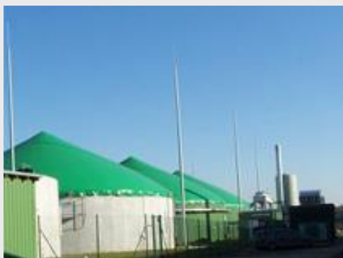
1,6 MW el biogas plant in Velgast, Germany
