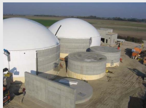
1 MW el biogas plant in Orth a.d. Donau, Austria
