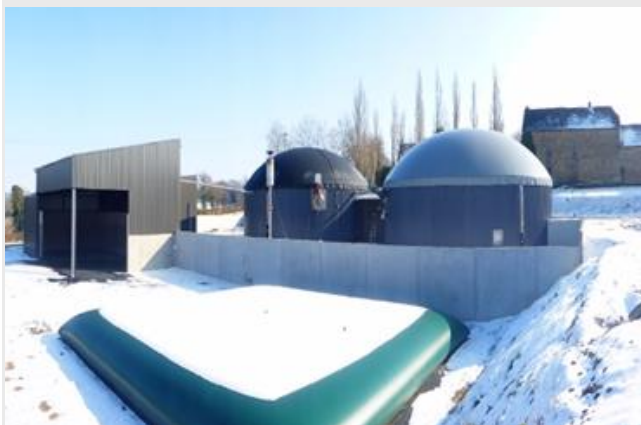
Biogas plant in Aveyron, France
