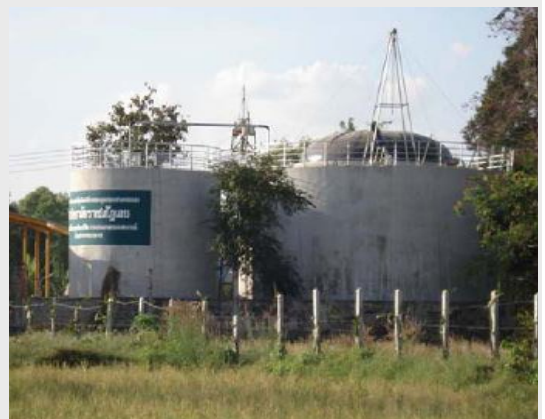
Biogas plant in Ubonthani, Thailand
