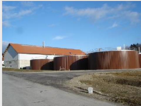
2 MW el biogas plant in Simbach, Germany
