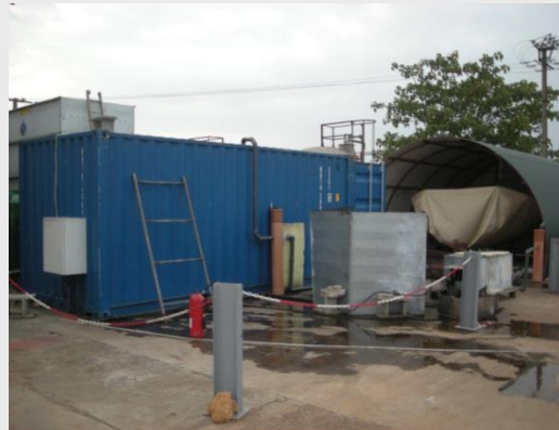
Container biogas plant (to test unconventional feedstock) in San Pedro, Ivory Coast
